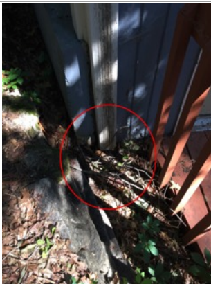
Missing downspout discharge
