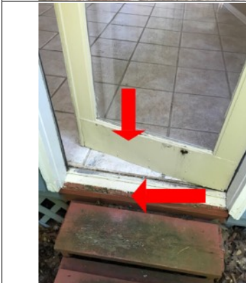
Door and sill plate show major signs of deterioration
