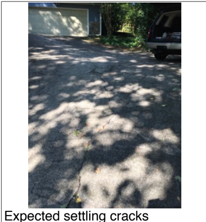
Expected settling cracks
