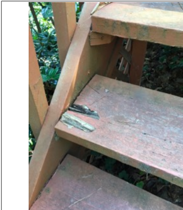
Deteriorated Front Steps
