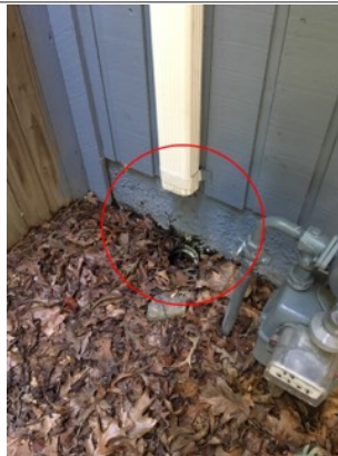
Missing gutter extension
