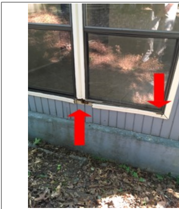
Deteriorated trim and siding
